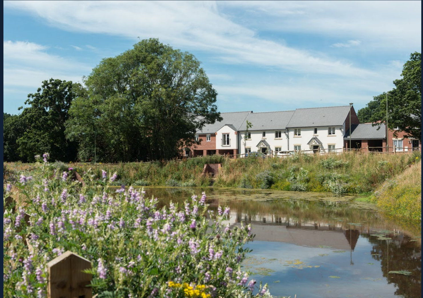
Image of previous Taylor Wimpey development with attenuation basin.
